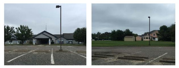
Parking spots south of the church can be replaced with porous asphalt to capture and infiltrate stormwater. Installing a rain garden in the turfgrass area southeast of the parking lot can capture, treat, and infiltrate parking lot runoff. A preliminary soil assessment suggests that the soils have suitable drainage characteristics for green infrastructure.
