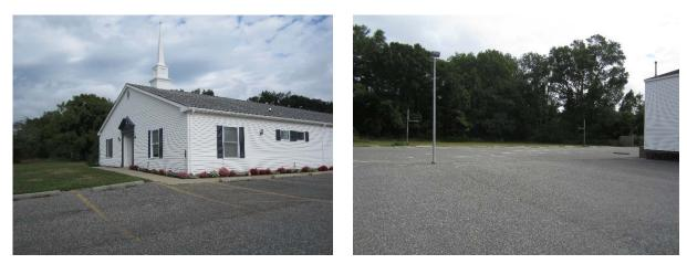
Parking spots in front of the building can be replaced with porous asphalt to capture and infiltrate stormwater. Installing a rain garden in the turfgrass area northeast of the church can capture, treat, and infiltrate parking lot runoff. A preliminary soil assessment suggests that more soil testing would be required before determining the soil's suitability for green infrastructure.
