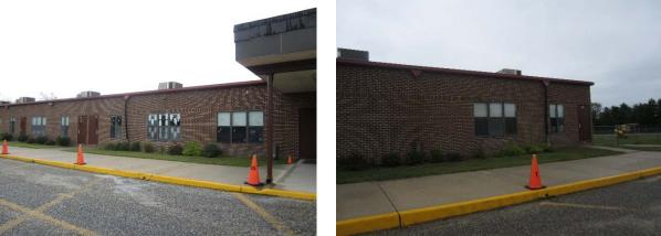
The sidewalk in front of the school can be replaced with porous concrete to capture and infiltrate rooftop runoff. A preliminary soil assessment suggests that the soils have suitable drainage characteristics for green infrastructure.
